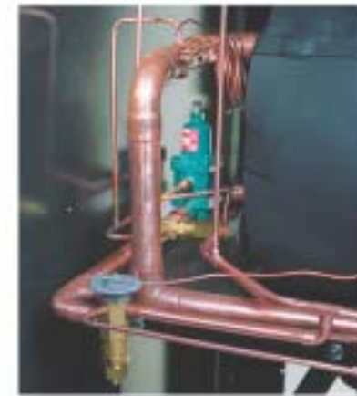
Refrigerant controls on models 1250 & larger
